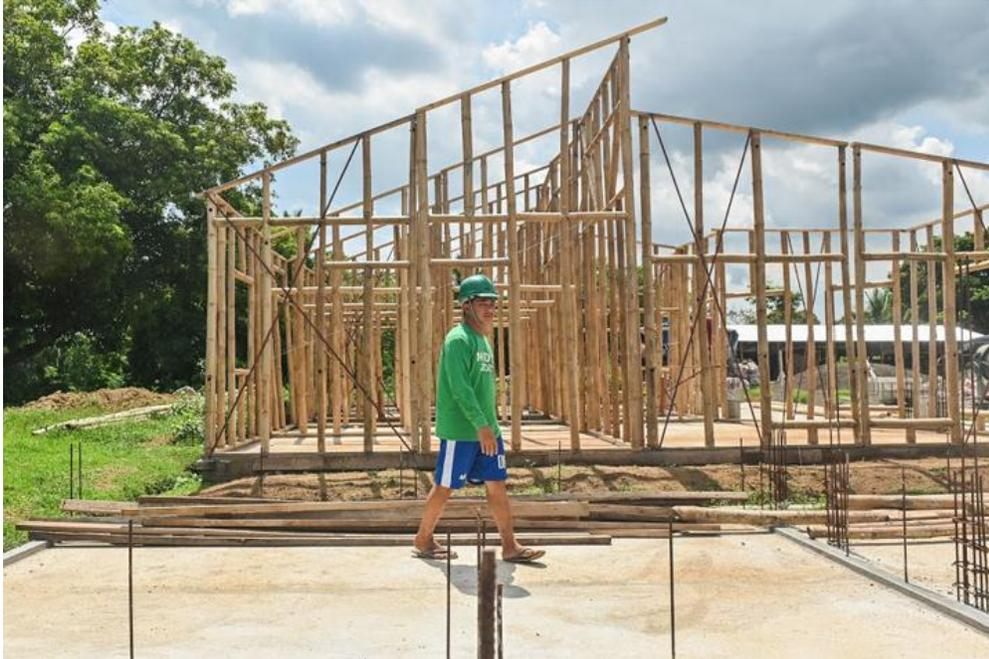
A worker passes by a structure using bamboos in building an orphanage with an innovative bamboo-cement technology in Batangas. Photos from Base Bahay Foundation Inc.
