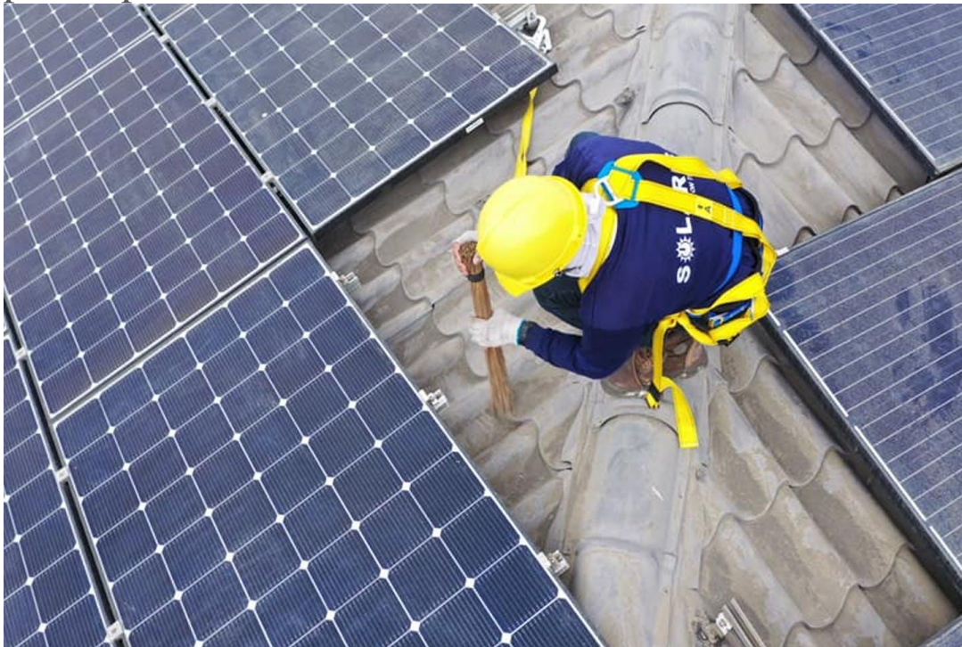
A worker cleans solar panels installed in a private residence in Manila, Philippines. Image: Solaric Corp.
