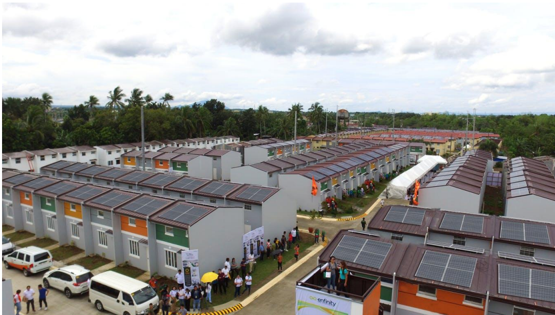
Solar panels installed in an affordable housing community in Sto Tomas, Batangas in the Philippines. Each 40 square meter house is equipped with a 1.2kWp solar panel. Image: Enfinity Imperial Solar Solutions
