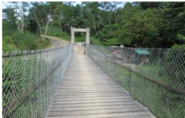
Connecting communities through the construction of bridges and roads.
